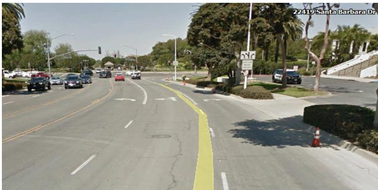
Figure 1: Manhole on Santa Barbara. Traffic control closes center lane.
