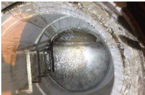
Manhole Before Install
