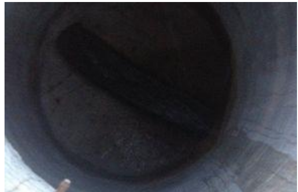
Manhole Before Install
